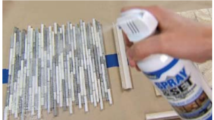
Be sure to apply a light coating (back-buttering) to mesh-backed tiles.
